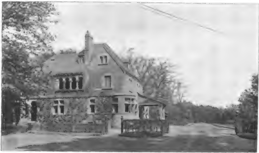
OFFICE ON MAIN THOROUGHFARE.
